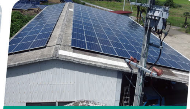
Project size: 104KW Site Location: Japan Finished Time: 2018 Project type: Trapezoidal Roof Mounting
